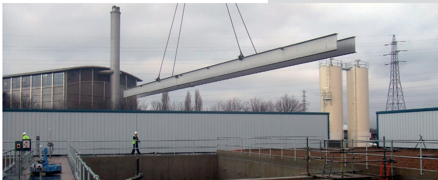
Figure 8: Installation of a pair of main beams
