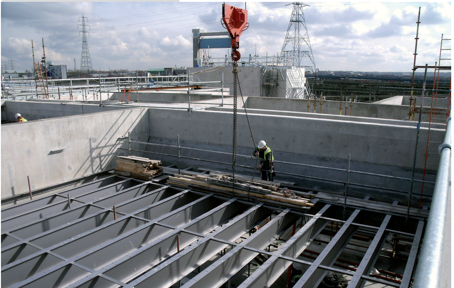
Figure 7: Completed lamella steelwork
